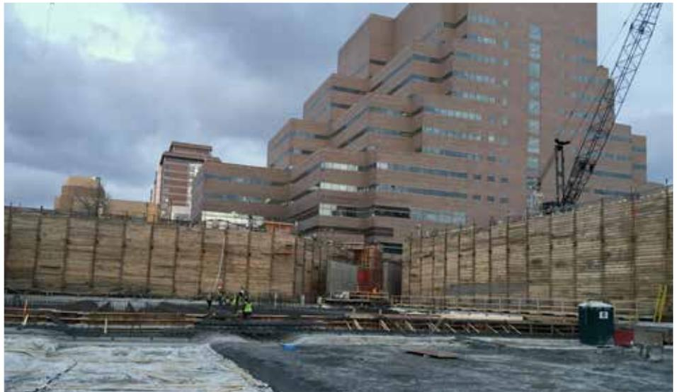
allowed the use of stock H-beam soldier piles in lieu of utilizing heavier WF-beam sections from a mill rolling. Grouted hollow bar anchors were chosen for the tiebacks due to their speed and ease of installation. Nucor Skyline's large stock inventory of multiple H-pile sizes and 52mm and 40 mm hollow bar anchors allowed construction to proceed immediately after the contract was awarded.
